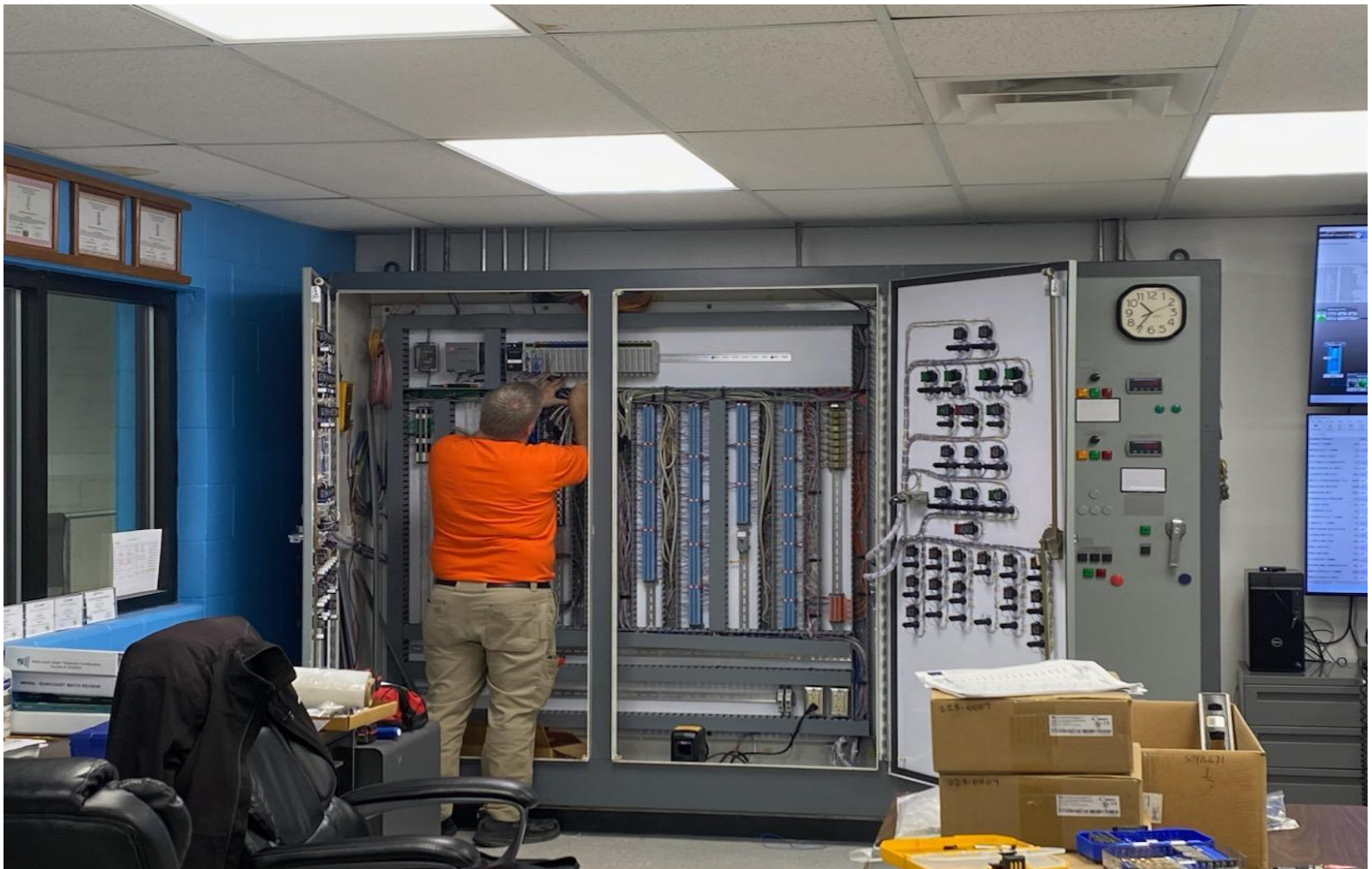
Micro Comm Replacing Programmable Logic Controllers in the WTP Lab
