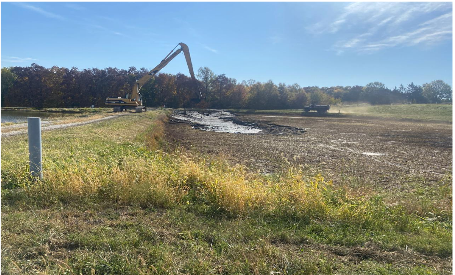
Contractor cleaning out south sludge lagoon
